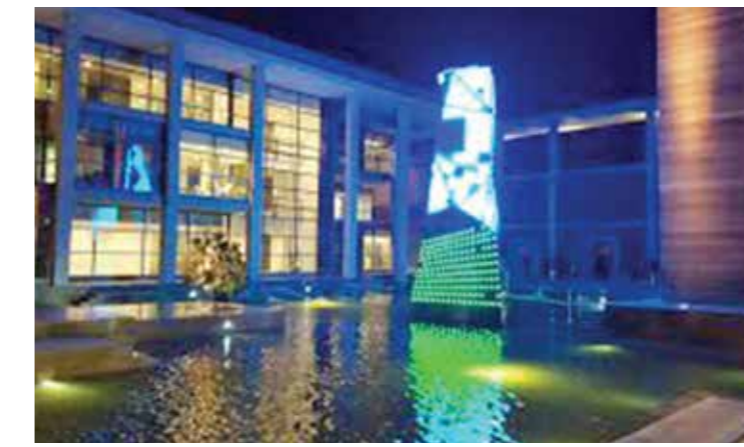
TELENOR HEAD OFFICE
